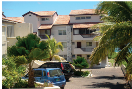
First floor Apartment Building
